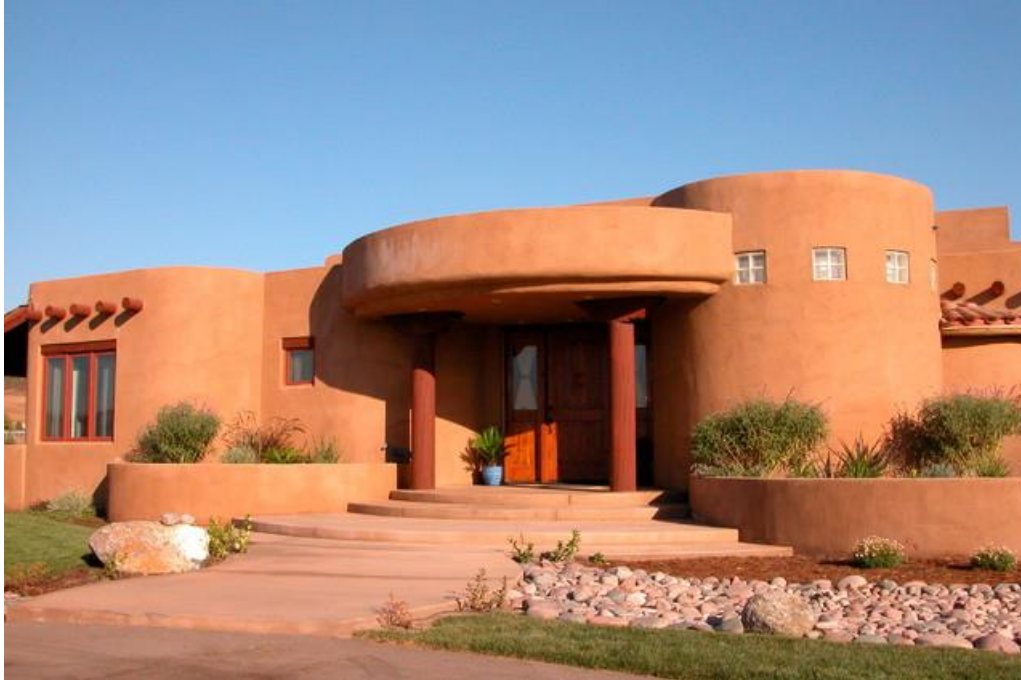
Figure 4-17 – Example of a modern adobe structure
