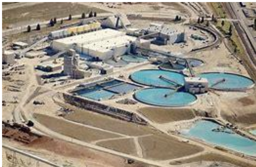
Figure 6-23 – Water treatment plant
