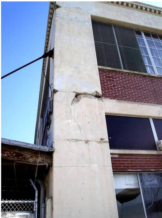
Figure 3-1 - Damaged concrete column, 2005 Hurricane Katrina
