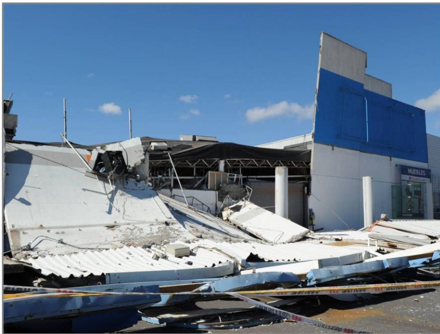
Figure 2-8 – Collapse of tilt-up walls, 2010 Chilean Earthquake
