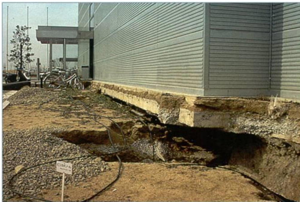
Figure 6-8 – Earthquake-induced settlement (Japan)
