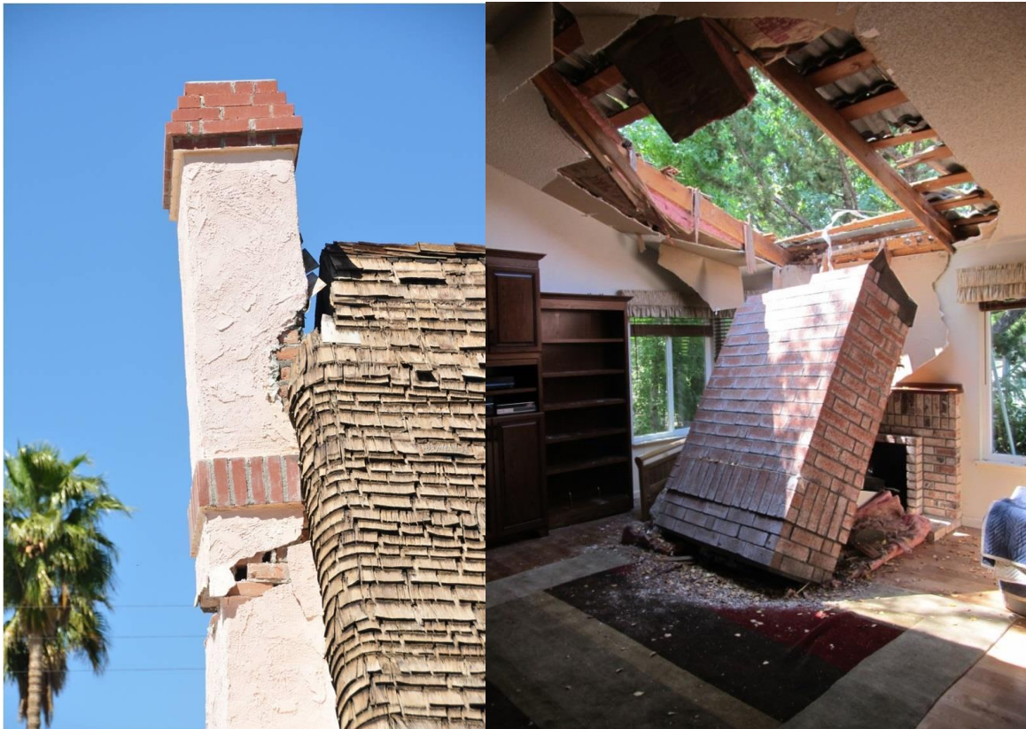
Figure 2-12 – Damaged chimneys
