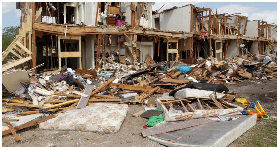
Figure 3-30 - Damage from West, TX fertilizer plant explosion, 2013
