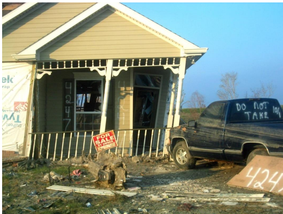
Figure 3-21 – Racking damage to wood frame building, 2005 Hurricane Katrina
