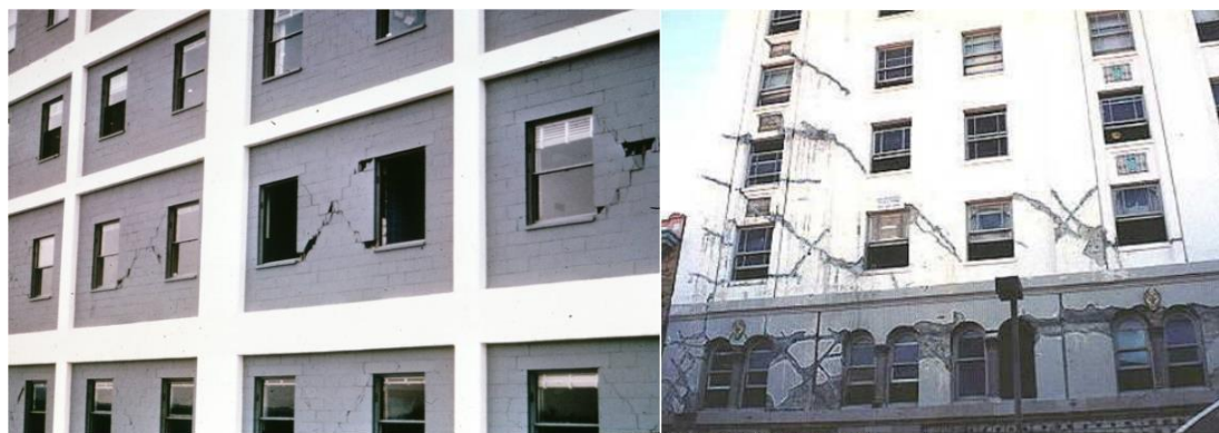
Figure 2-2 – Shear cracking
