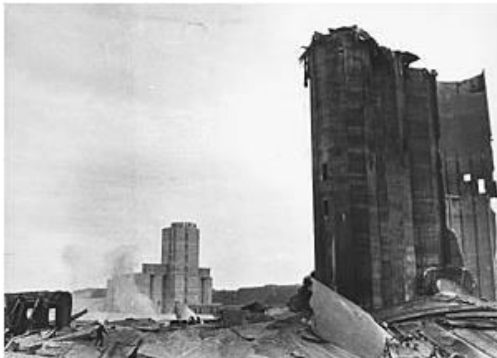
Figure 3-25 – Explosion – damaged granary
