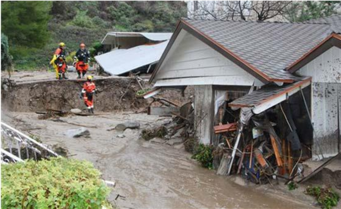
Figure 3-22 Debris flow damage to house
